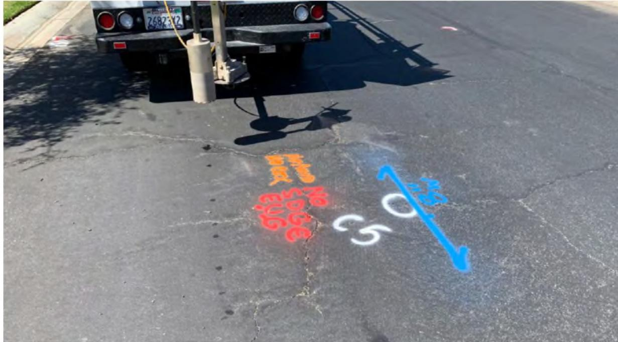
Photo 3: Coring location C-5. Surface contains low to medium-severity longitudinal and transverse cracking.
