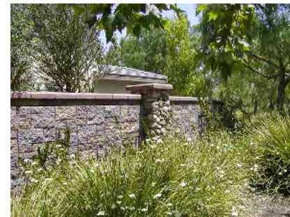
split-face block and stone
