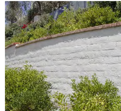
sacked slump block
