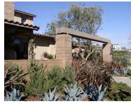
slump block & timber
