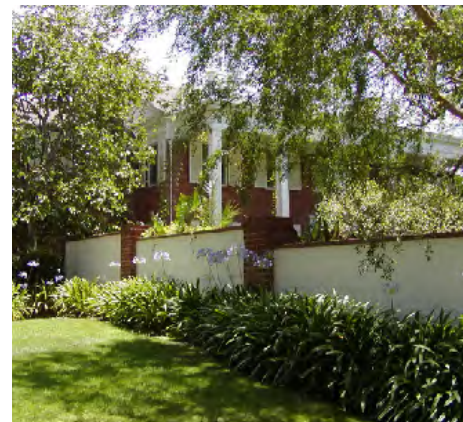
stucco and brick
